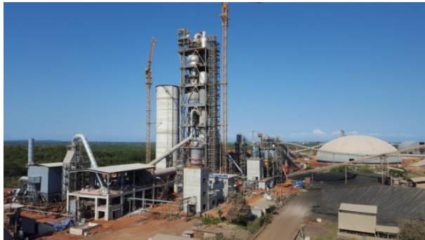
CBMI project construction
